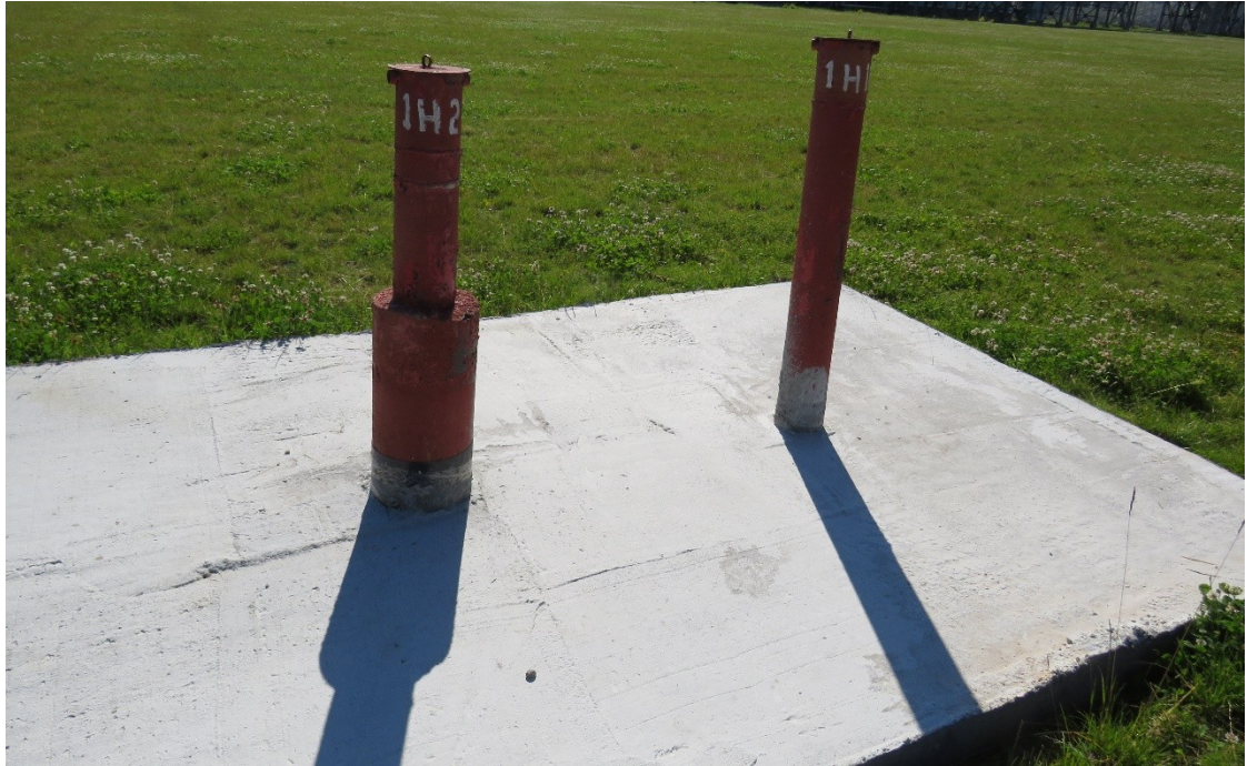
Figure 8.6 - Piezometric well cluster
