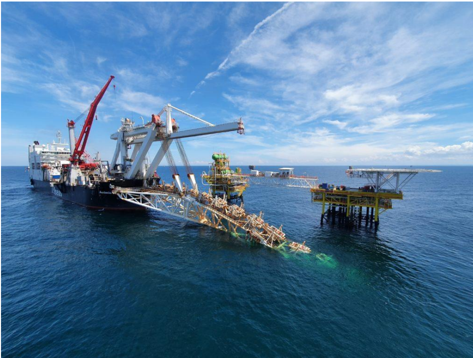
Figure 14. Laying of pipelines from a specially equipped vessel (Allseas).
