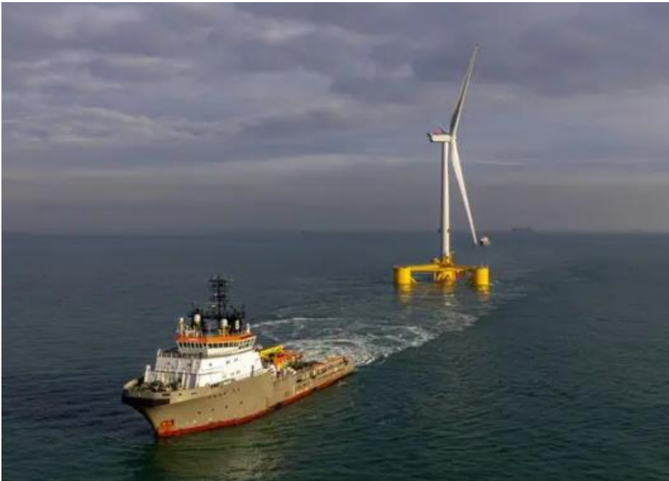
Figure 13. Towing of a wind turbine with a floating foundation (Tomic, Bartolomej 2020).
