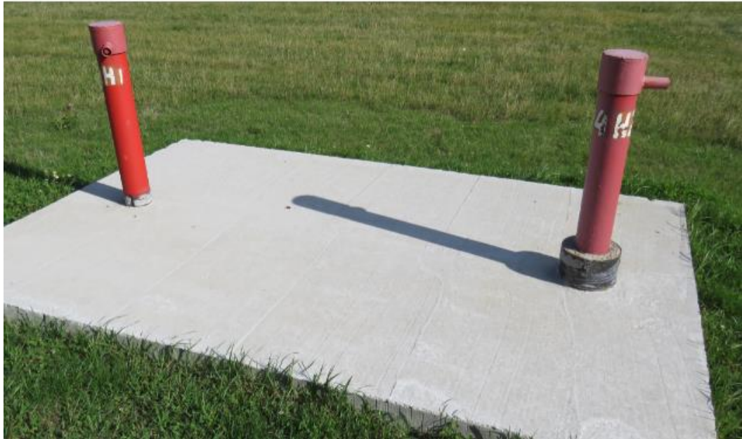
Figure 8.6 - Piezometric well cluster
