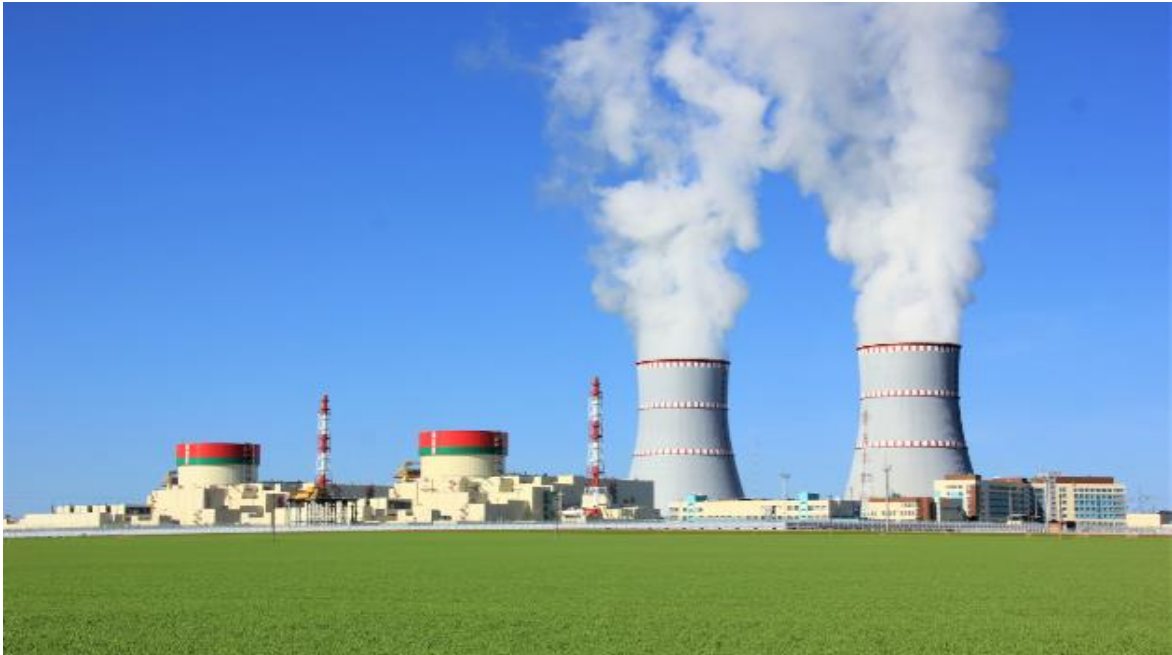
Figure 2.1 - Belarusian Nuclear Power Plant
